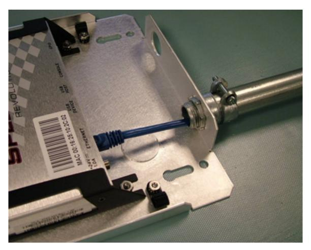
Figure C.7 A squeeze connector for the larger ¾ inch conduit tubing size. The connector has a nut and threads sized for the ½ inch conduit hole.
